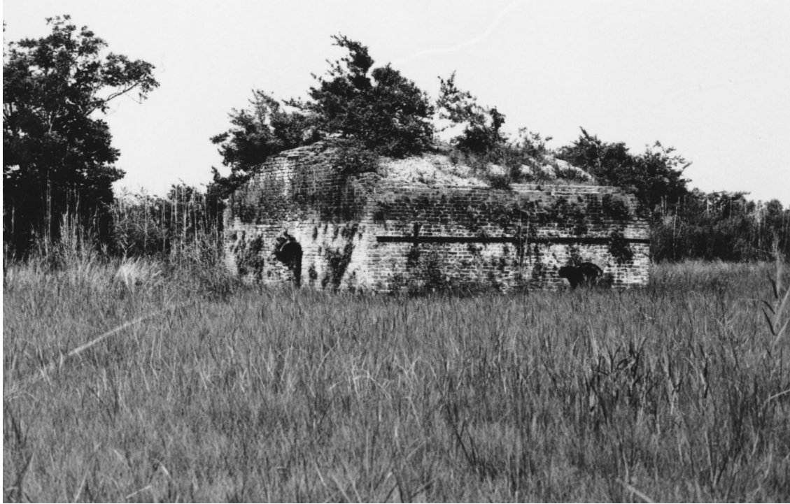
Figure 2-9. Ground view of powder magazine at Battery Bienvenue looking to the east, June 10, 1976 (Gagliano et al. 1978).
